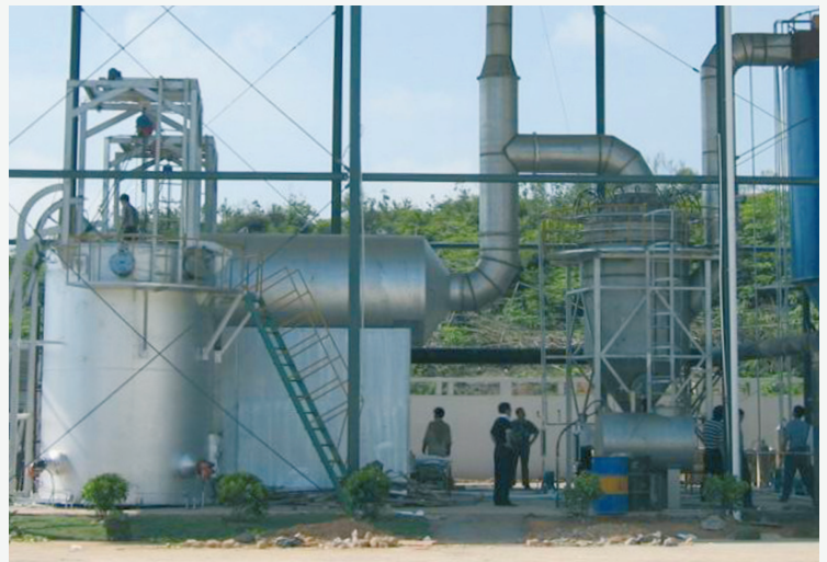
LFRY-8 medical waste incinerator with a daily disposal capacity of 8 tons located in Jiangmen
